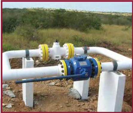
6" 600 ANSI with 6" bypass line Tamaulipas, Mexico
